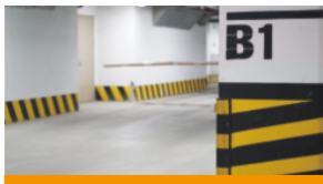
Parking Control And Charge Management
